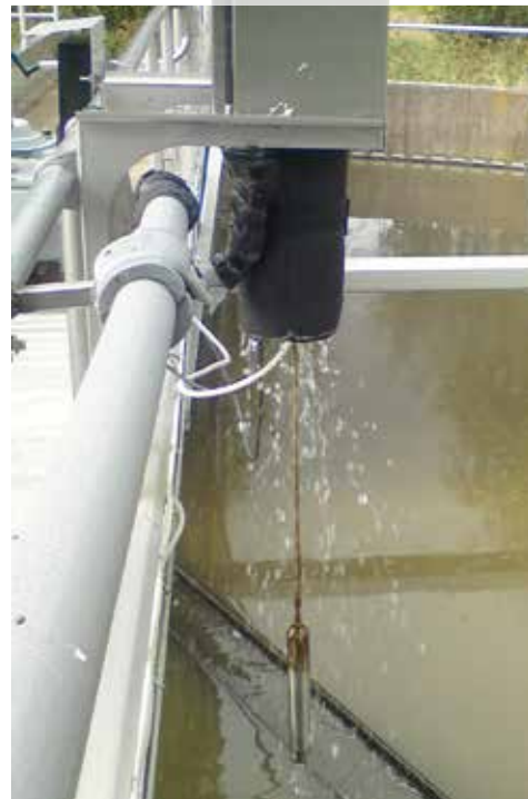
CBX with mounting assembly for easy attachment to handrail. Automatic flushing system of cable and sensor after each cycle.
